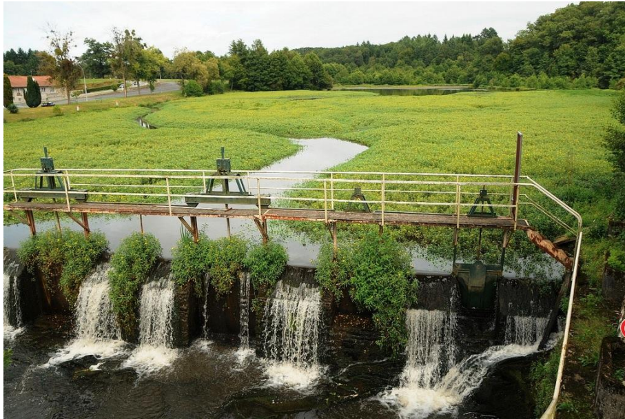
Photo 1: Clogged floodgate by Ludwigia peploides in France.
