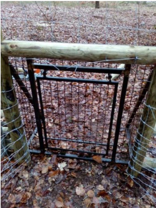
Figure 6 – Unidirectional "cat flap" door 1m high
