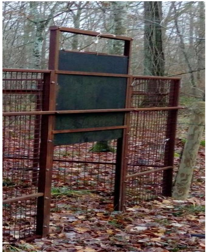
Figure 7 – Guillotine door in plywood panel
