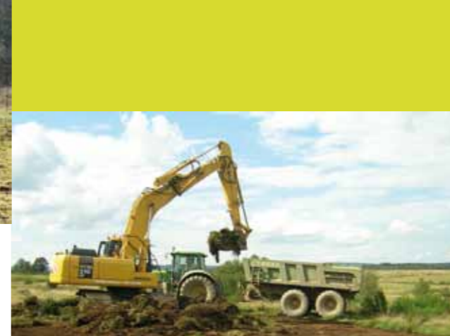
Removal of plaggen
