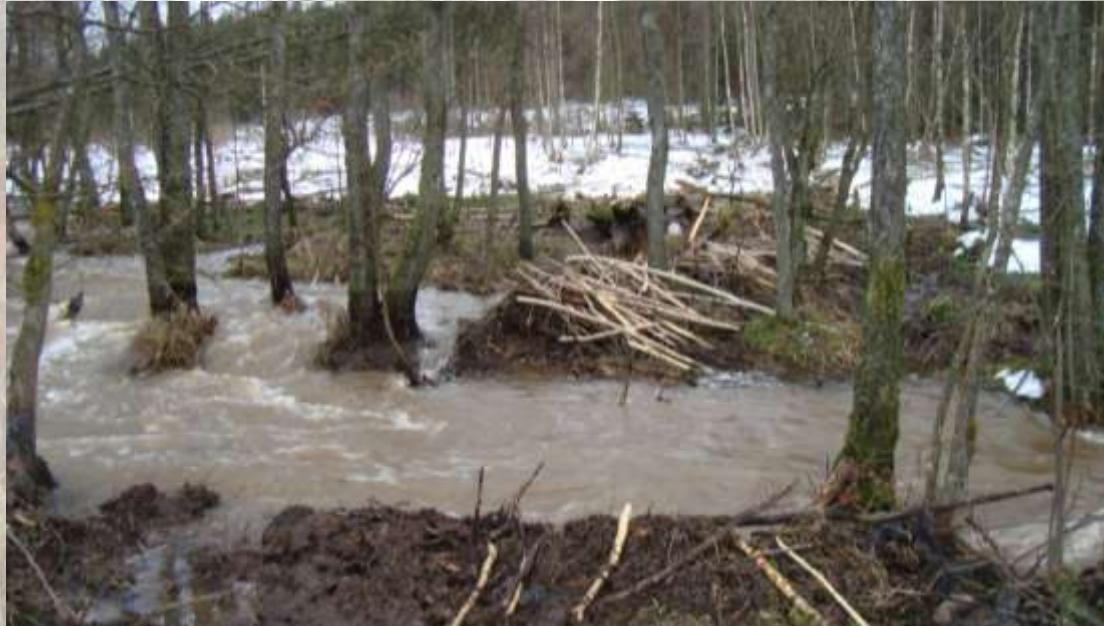
Failure of beaver dam 2.17 in January 2011; the wood debris (middle) are rests of dam material removed from the stream bed by municipal workers (recent traces of machinery) to protect a road (behind the photographer) from flood. The dam was destroyed at high water level, probably the maximum of the flood, as can be observed from the extent of the snow-free area and from humidity on standing trees.
