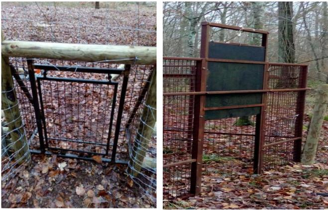
Figure 6 – Unidirectional "cat flap" door 1m high
